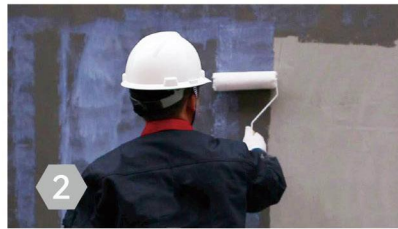
2 Apply primer to the desired surface.
