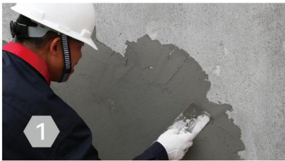
1 Inspect surface and eliminate potential risk.
