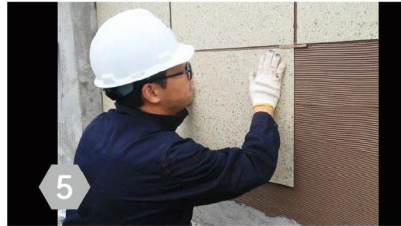
5 Install Flexible Stone panels.
